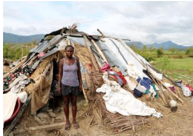
A resident in Tiburon commune stands in front of her collapsed home. © Medair / Nath Fauveau
